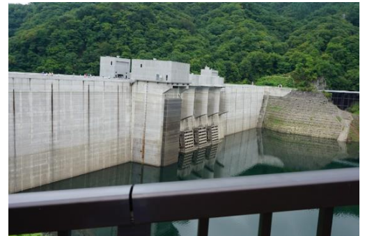
upstream view of the dam
