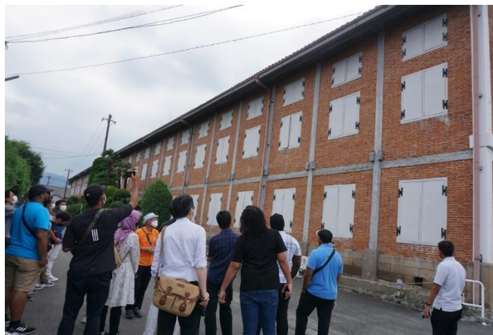
Tour talk on the front view of east cocoon warehouse
